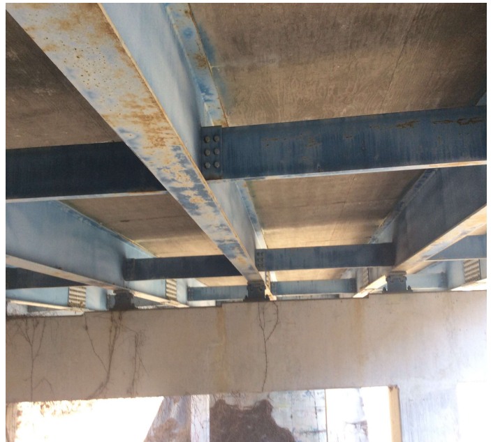
PHOTO 2 Description All girders have paint is chalky and they have some light rust to bottom and top flanges.
