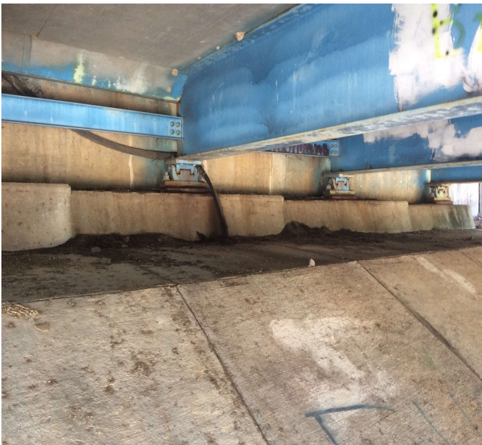
PHOTO 1 Description Bearings 1 - 3 at abutment 1, pack rust to masonry plates.
