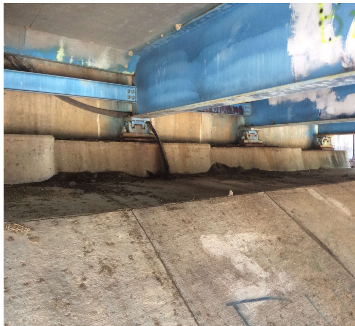
PHOTO 1 Description Abutment 1, joint material is hanging down on top of the cap and there is dirt and debris on the cap.
