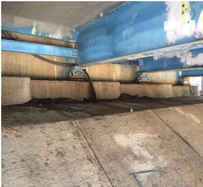
PHOTO 1 Description Bearings at abutment 1 pack rust
