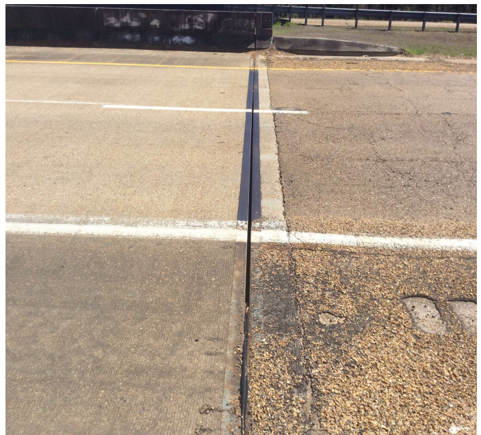
PHOTO 2 Description Joint material missing abutment 1, from 2' past the outside white line to 1' past C/L, over bearings 1 - 3.
